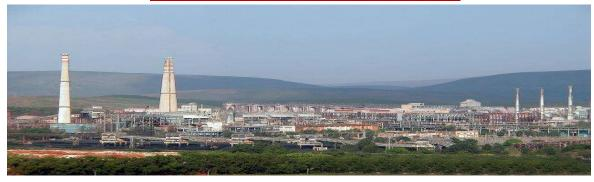
The **Alumina Refinery Plant** of NALCO is situated in the picturesque valley of Damanjodi. The energy efficient Refinery Plant has four parallel streams of equal capacity. The annual production capacity of the plant is 21 lakh tons.
