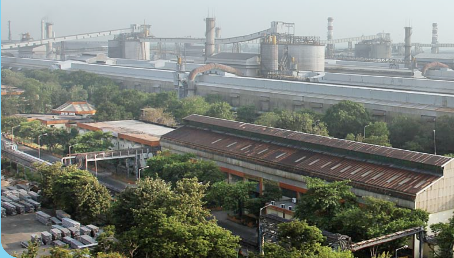
Panaromic view of NALCO's Smelter at Angul, Odisha
