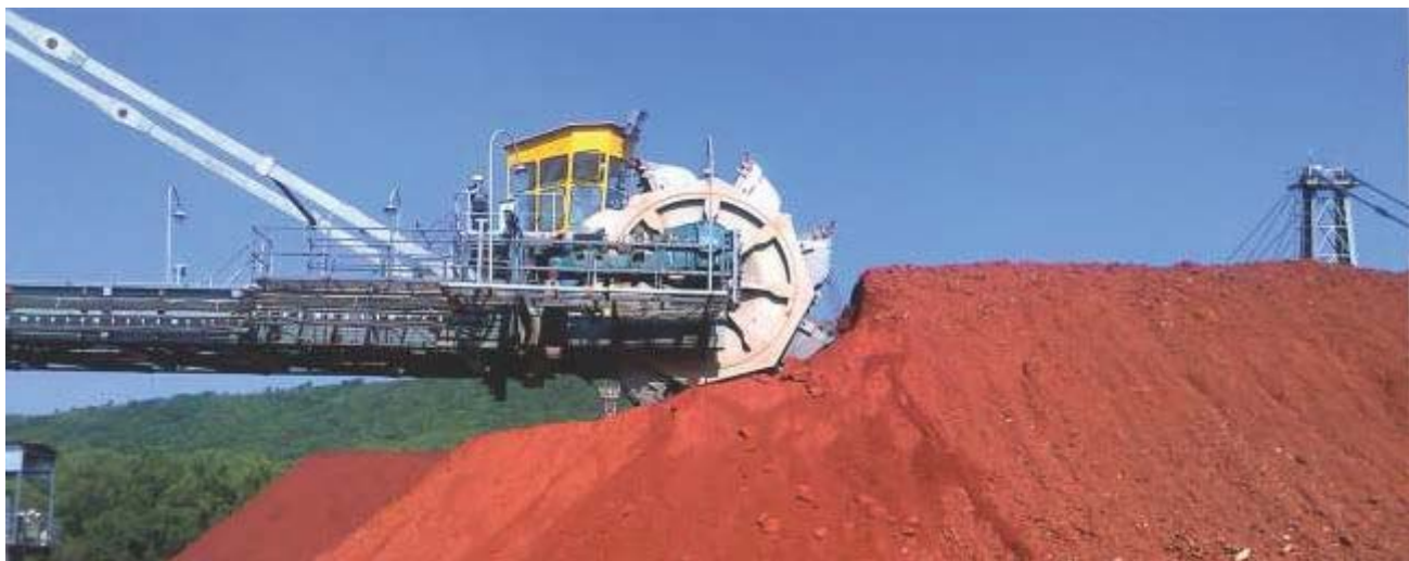
Reclaimer in operation at M&R complex, Damanjodi
