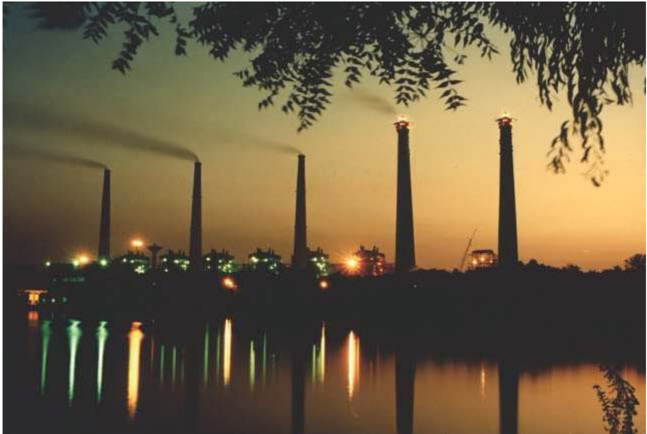
Panoramic view of Captive Power Plant, Angul
