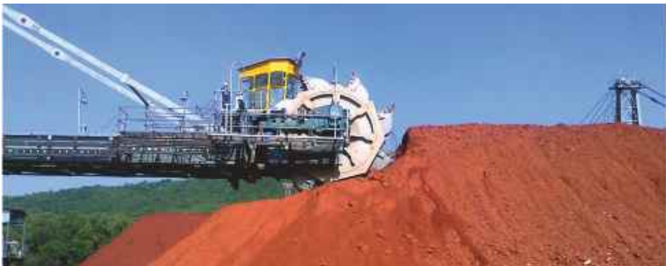
Reclaimer in operation at M&R complex, Damanjodi
