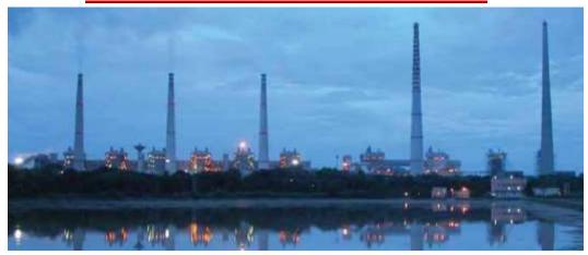
Close to the Aluminium Smelter at Angul, a Captive Power Plant of 1200 MW Capacity has been established for firm supply of power to the Smelter. The coal demand of the Plant is met from a nearby mine of Mahanadi Coalfields Limited. The plant is also connected with the State Grid for sale of surplus power.
