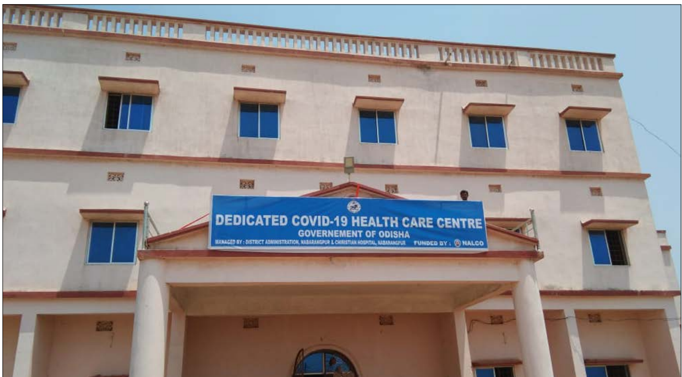
NALCO Funded 200 bedded dedicated COVID-19 hospital at Nabarangpur
