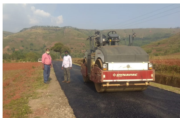
CSR project- construction of road in periphery area
