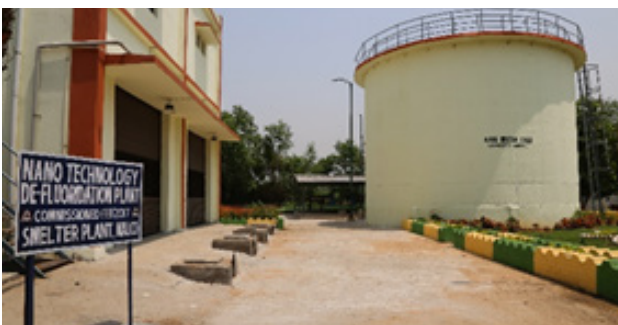
Nano-technology DF plant at Smelter
