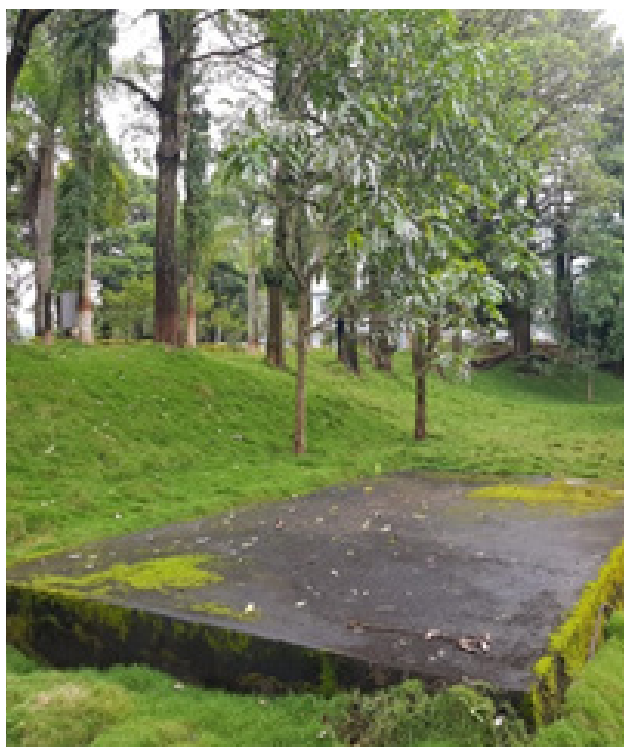
Re-charge well of roof-top rain-water harvesting at Refinery
