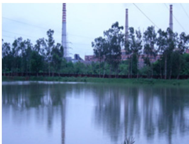
Rainwater reservoir at CPP
