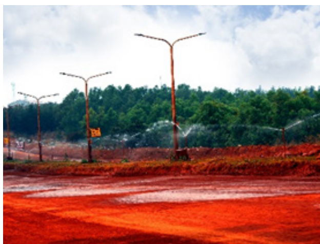
Water sprinkling in mines haul road
