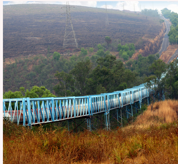
14.6 km long single flight belt conveyor from Mines to Refinery
