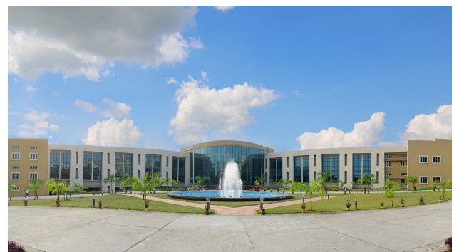
NALCO R&D centre NRTC at Gothapatna, Bhubaneswar
