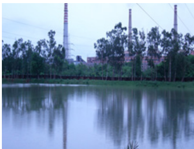
Rainwater reservoir at CPP
