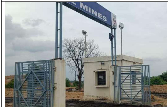
Camera to monitor tarpaulin covering
