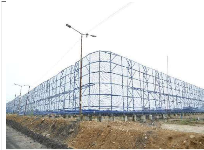
Wind Screen around coal stock yard
