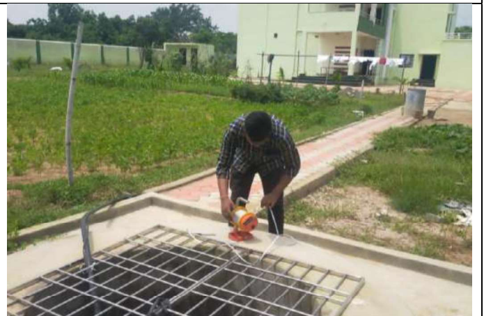
Piezometer for water level (village)
