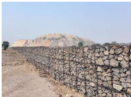
Stone retaining wall around OB dump
