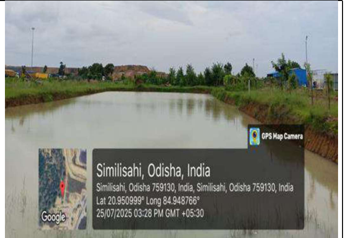
Rain Water Harvesting Pond
